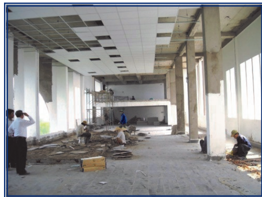
Library under construction at Tim Lanh Bible School in Saigon, Vietnam
